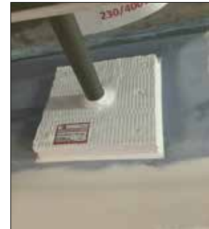
The finished seal.
