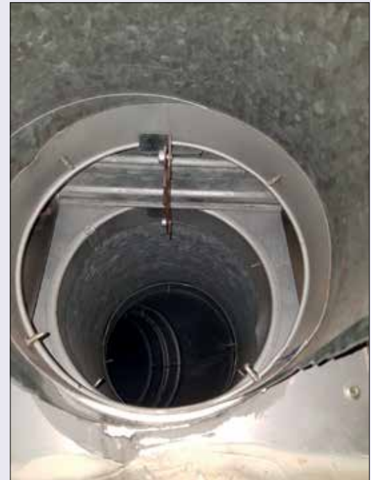
An example of poor installation illustrating self-tapping screws used to fix the galvanised duct to the fire damper pigot.
