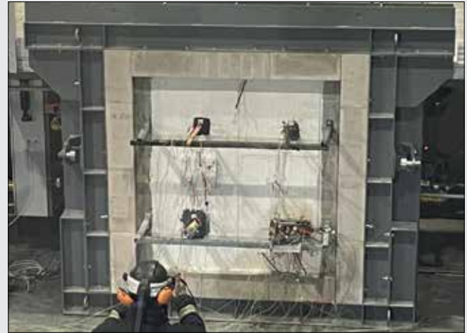
iv. After the test; external (non-furnace) side
