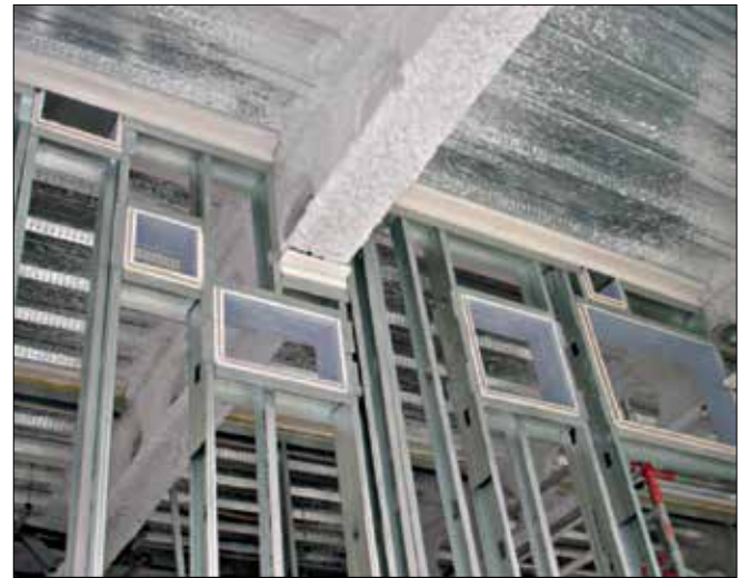
Prepared openings for services in a dry-lined partition fire wall.
