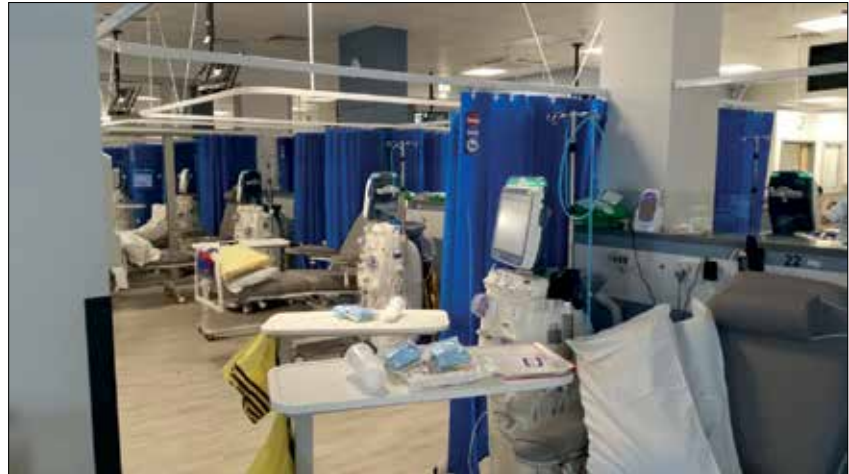
A Renal Unit needs to be robustly protected in terms of critical care continuity.
