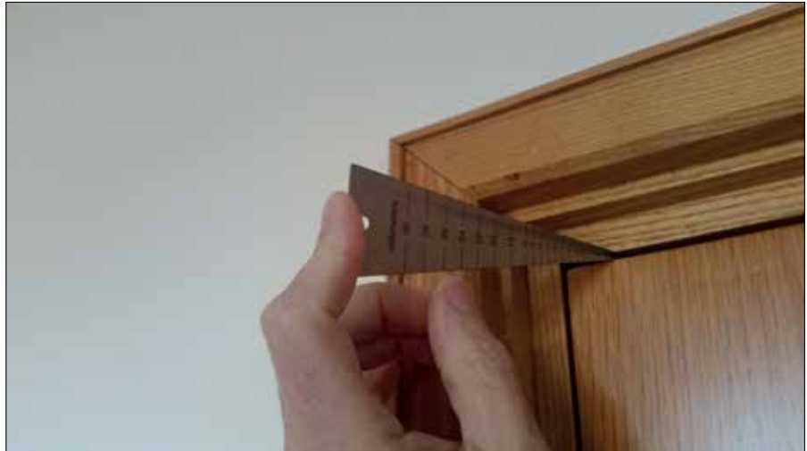
Checking the top edge of a door leaf during a Type 1 inspection. Image courtesy of Golden Thread Fire Delay
