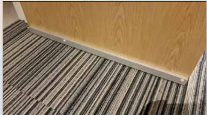
A door leaf bottom edge, fitted with a drop down seal.
