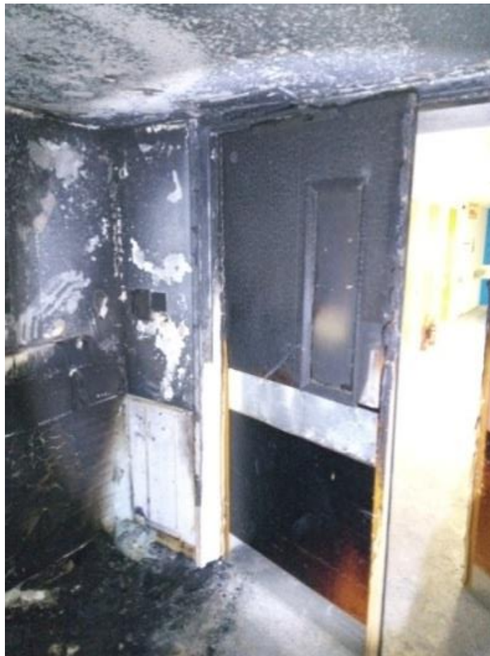
Photo 5 - this shows the fire damage at the seat of the fire how fire doors offered protection
